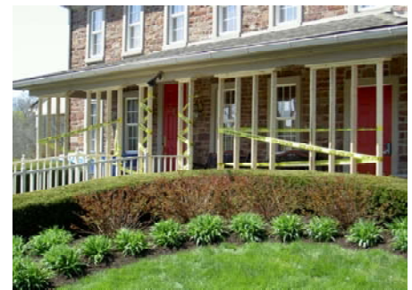
Repairs to columns on porch of Clubhouse
